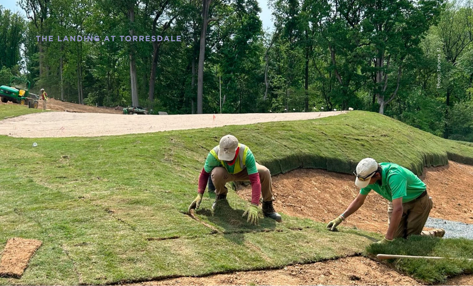
Tahoma 31 sod was laid on 80,400 square feet of green surrounds and slopes
